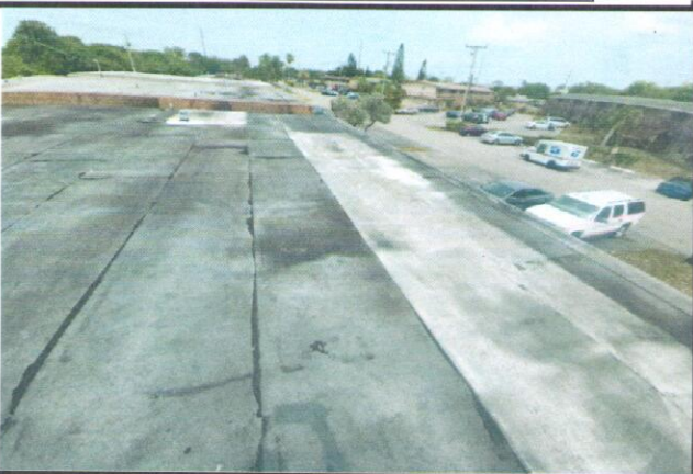
Flat Roof Covering (Need New Flat Roof)
