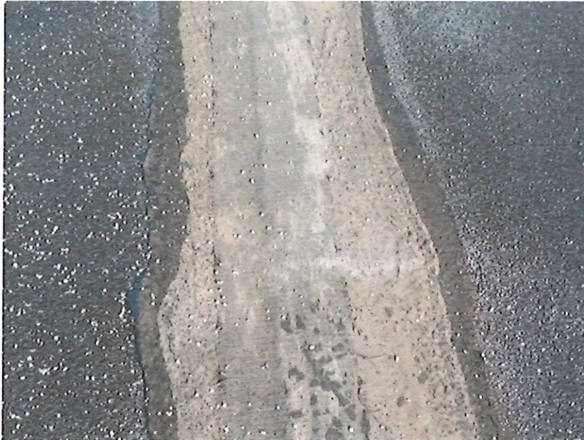
cracking on existing roofing material
