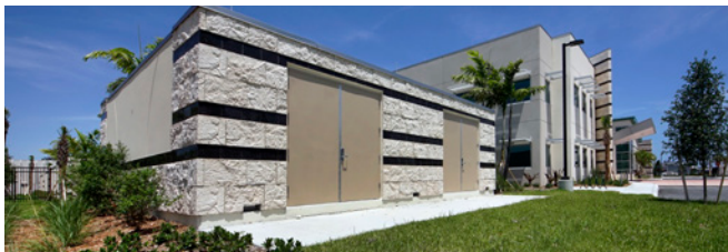
Example of mechanical equipment screened from public view
